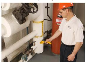
Darryl Dylla, HVAC/Power Plant Manager, uses a Fluke 62 Infrared Thermometer to check steam traps throughout the HVAC system.
