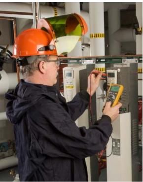
Jim Murphy, Electrical Foreman uses the Fluke 179 DMM to look at low voltage signals in the newly installed VFD for the 40+ year old steam system.
