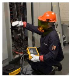
Rolf Zoeller, Electrician uses the Fluke 1735 Three-Phase Power Logger to do load studies on the hospital's electrical systems. Keeping close tabs on these systems helped the hospital achieve its ENERGY STAR rating.
